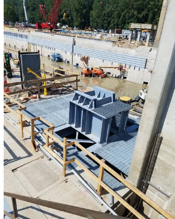
New gate machinery base
