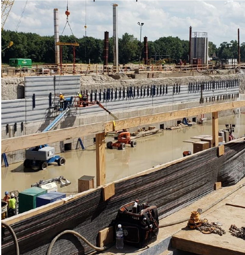
Vertical concrete pre-cast panel installation
